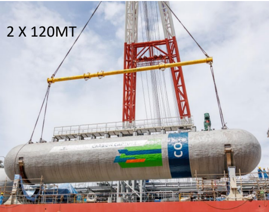
11 Dec 24 – LCO 2 Tanks Installed
